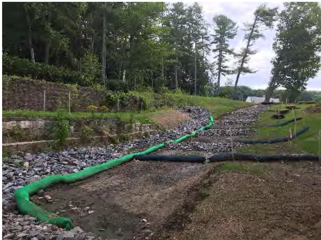
Fig 16: Slope above manhole at Gundalow Landing/east side of the bay. Viewing northeast. (07-27-20).
