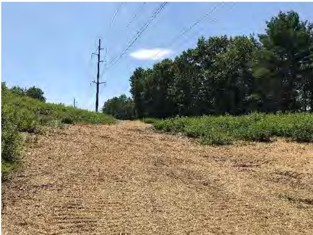
Fig 2: Access road between Strs. 45 and 46 mulched and seeded. Viewing south. (07-27-20).
