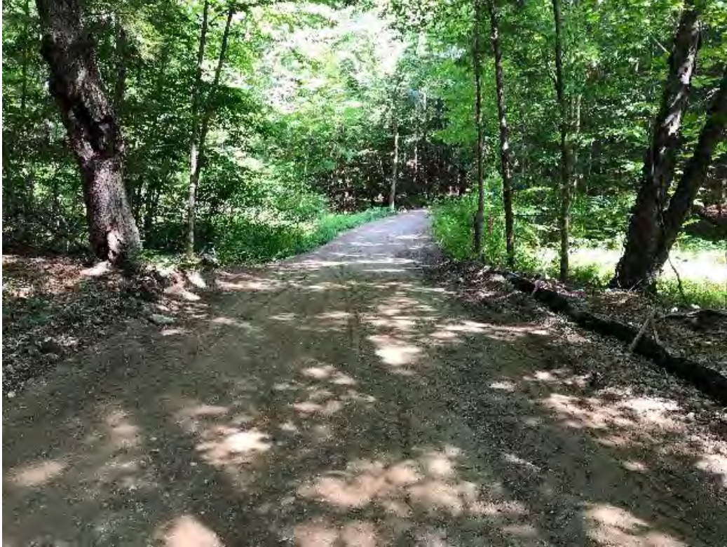
Fig 5: Access road to Strs. 9-18 off Route 4 was re-graded. BMPs along access road to be removed. Viewing east. (07-27-20).
