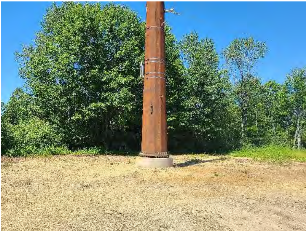
Fig 10: Str. 48 work area mulched and seeded. Viewing west. (07-29-20).
