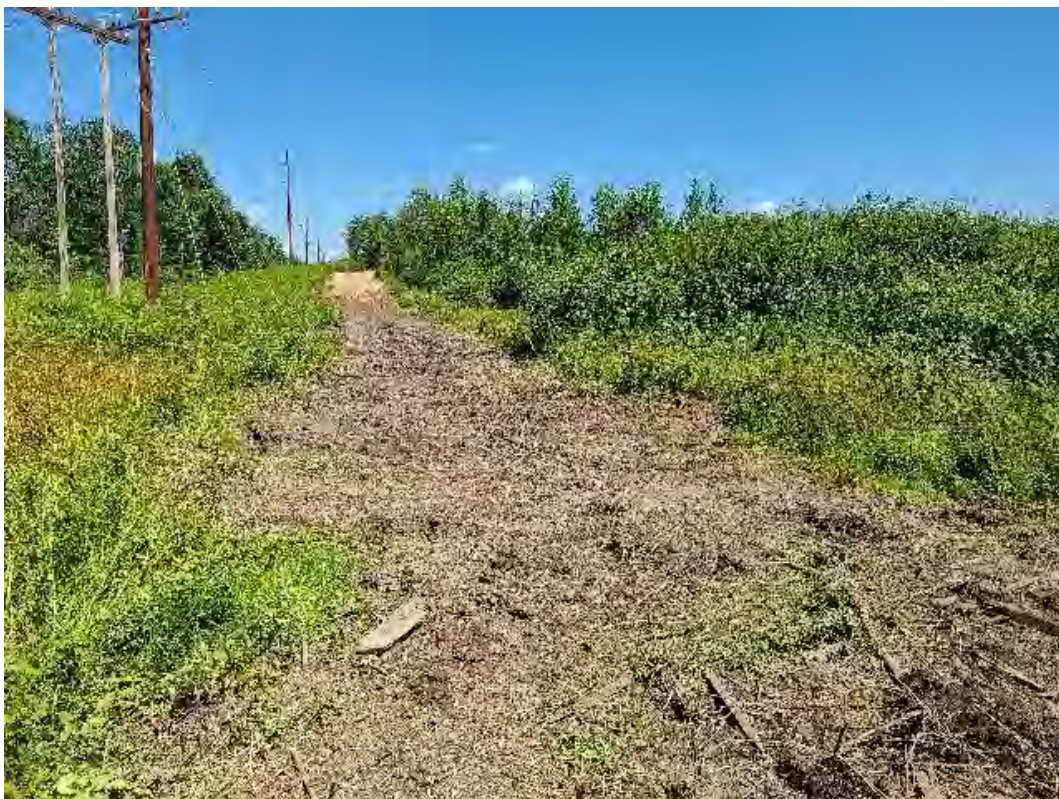
Fig 8: Timber mats removed from access road between Strs. 47 and 48. Viewing north. (07-29-20).
