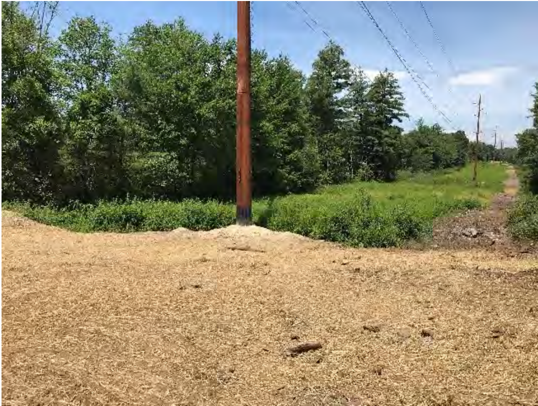
Fig 1: Str. 45 work area mulched and seeded. Viewing northwest. (07-27-20).
