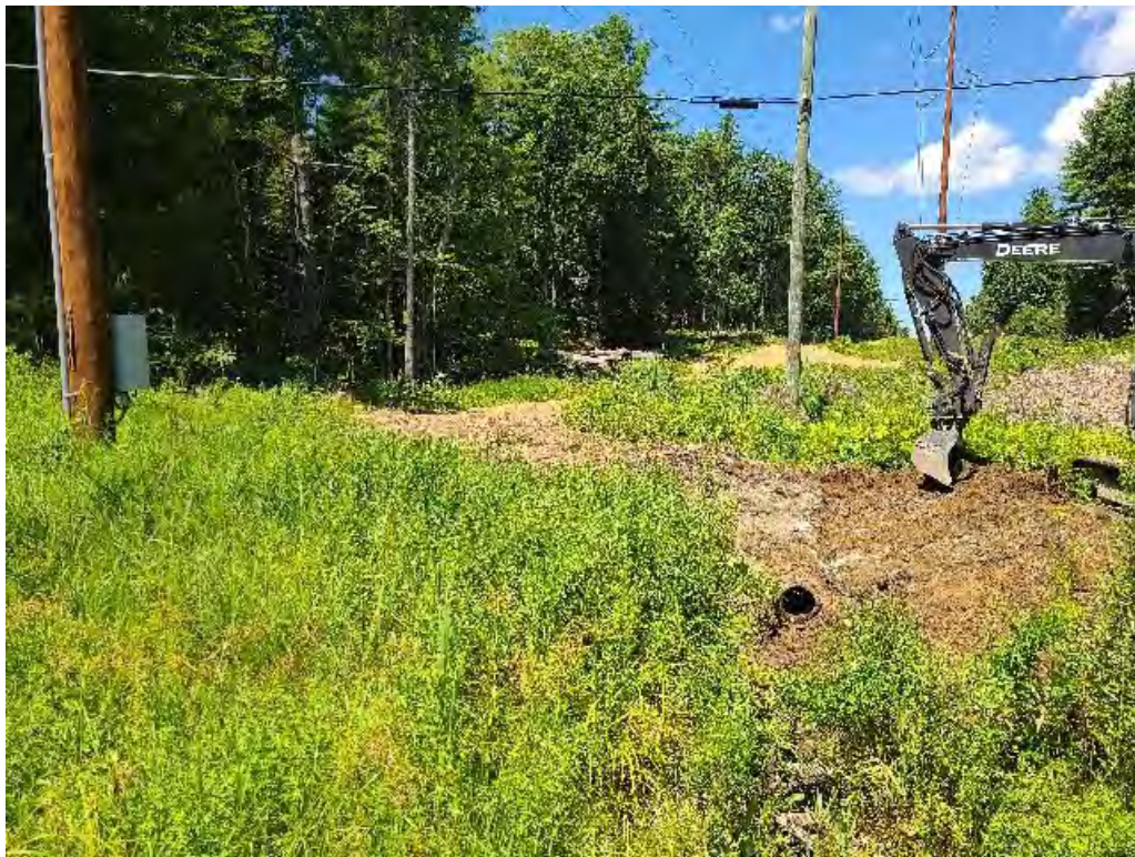
Fig 6: Replacing culvert off Durham Point Rd. Viewing northwest. (07-29-20).
