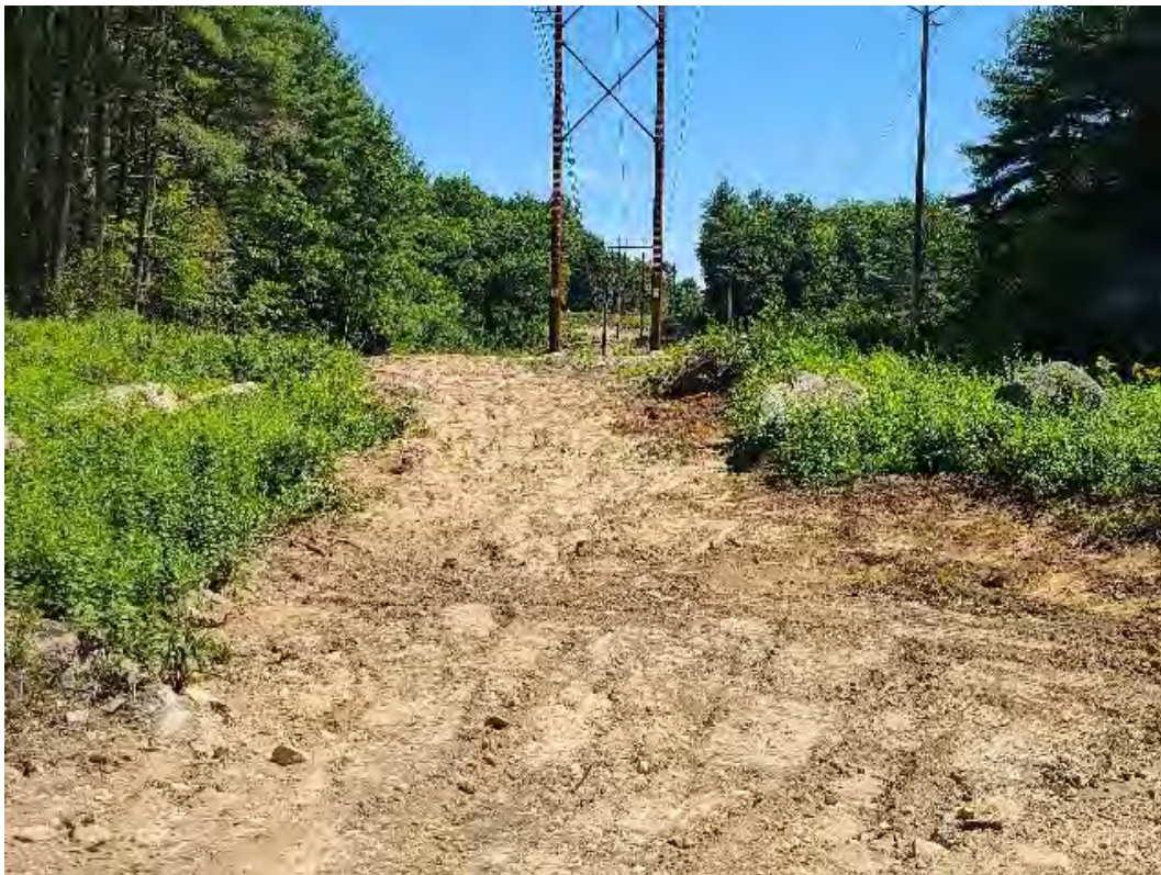
Fig 12: Restoring access road between Strs. 55 and 56. Viewing northeast. (07-29-20).
