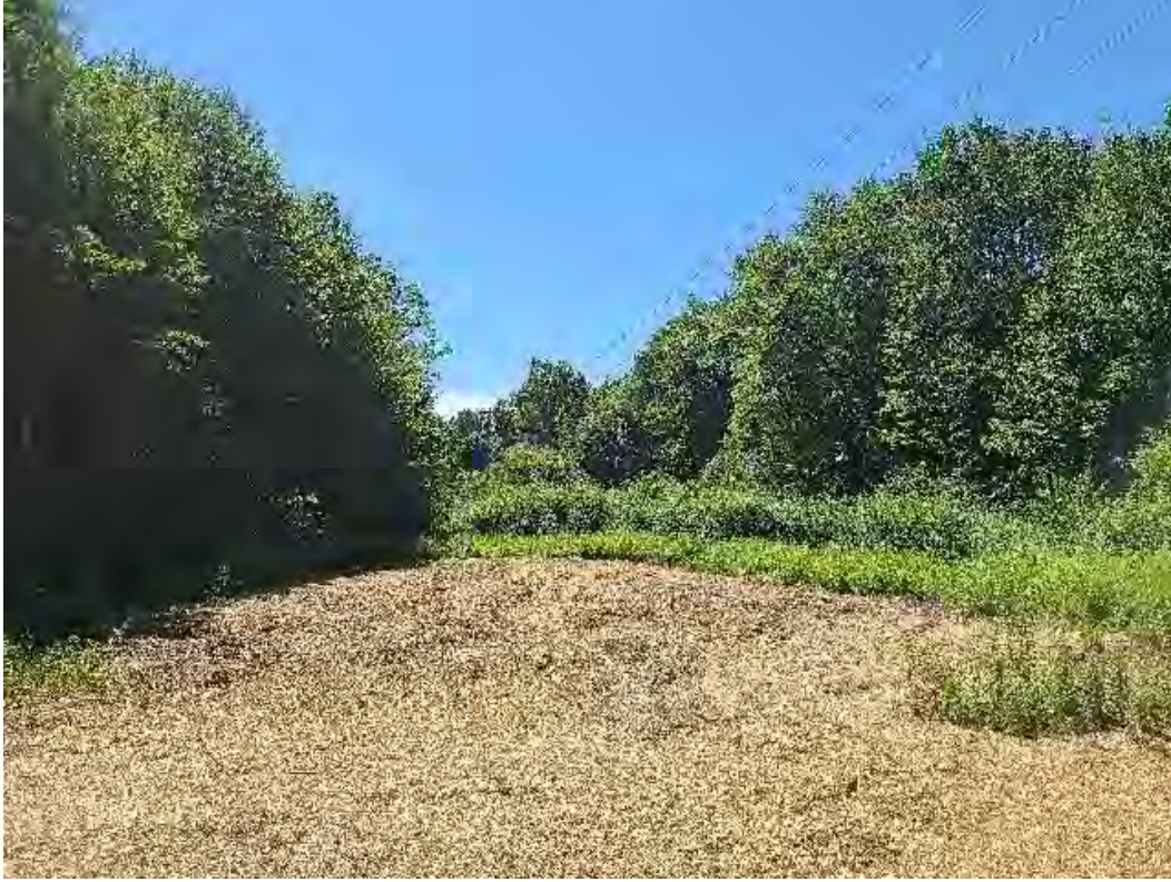
Fig 9: Dewatering basin at Str. 48 regraded, mulched and seeded. Viewing south. (07-29-20).
